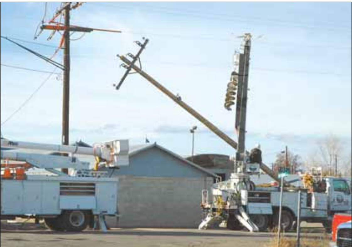
Idaho Power contractor ramps up Homedale’s capacity A crew from Meridian-based H&H Utility Contractors Inc., tilts a power pole into place last week at the corner of West 1 st Street South and West Wyoming Avenue. The work was part of an Idaho Power project to bolster the capacity of power lines along West 1 st Street from Wyoming to California avenues.
